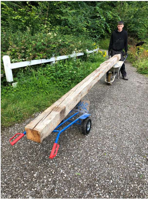
One of the main beams being brought to site.
