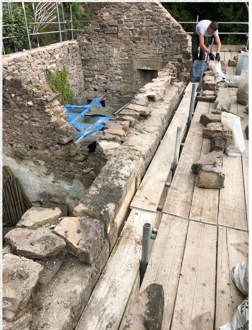
The top three courses of the front and rear walls were dismantled and rebuilt.
