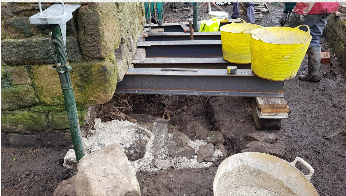
Underpinning the cottage. The corner of the building was supported by several steel beams until a new foundation of stone was built.
