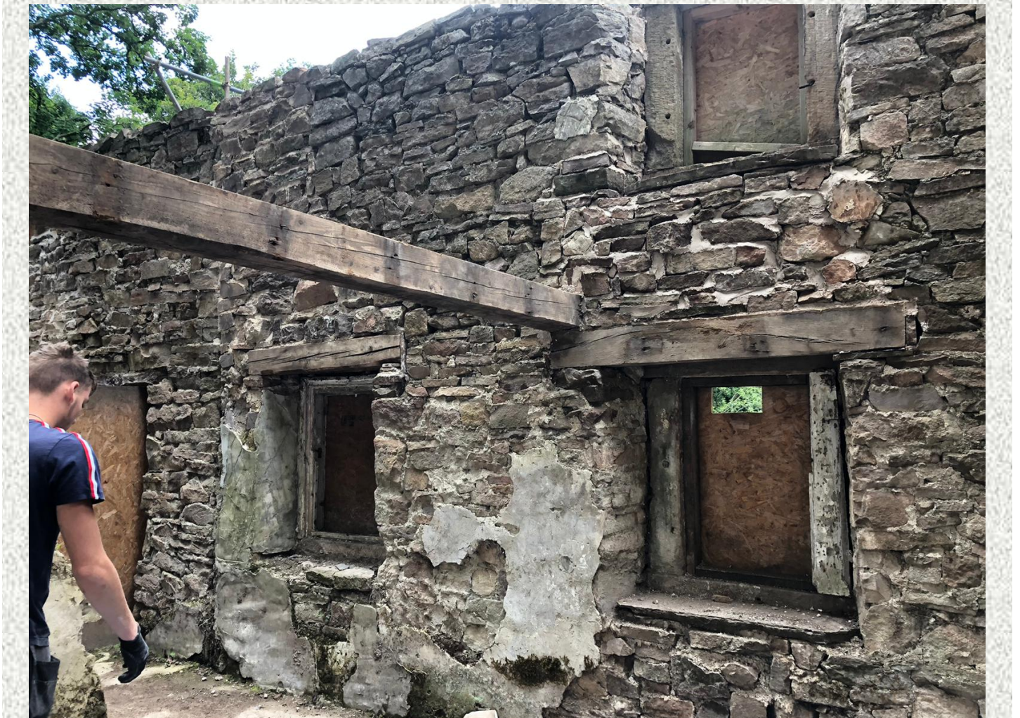
The two main beams installed.
